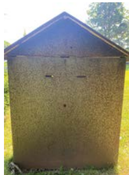
Original metal pill box used at the Mounds club provided slots for view and rifle to extend out.
