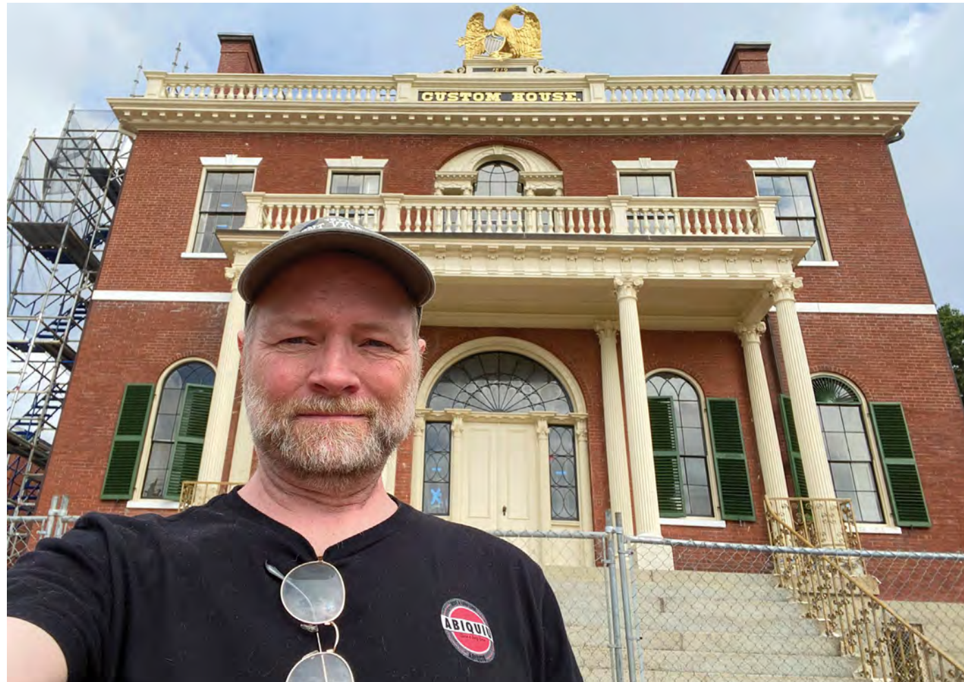
There was a Custom House in Salem since 1649, where taxes were paid on imported goods, first for the British Government, but after 1789 for the newly formed American Government. This iteration was constructed in 1819.
